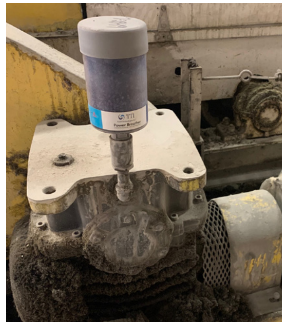
Figure 6. TTI Power Breather Installed
